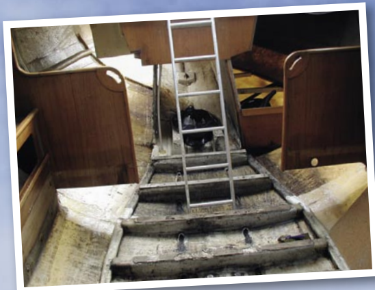
Almost everything had to be stripped out inside
