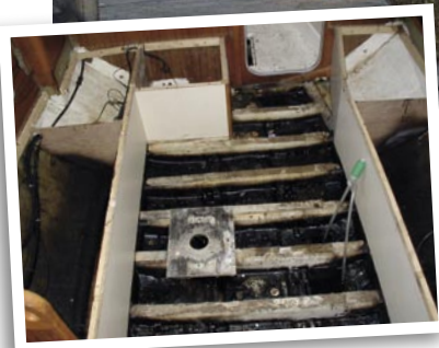
Elmarleen's bilges were full of oil from a ruptured diesel tank
