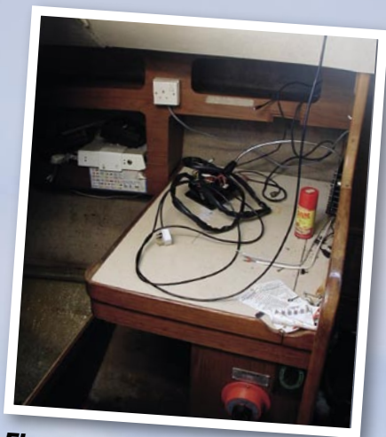
Elmarleen's electronics needed to be replaced
