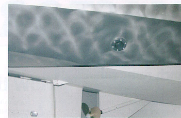
whether above or below the water. Also, as with a steel hull, condensation is a problem and the hull can be noisy.
